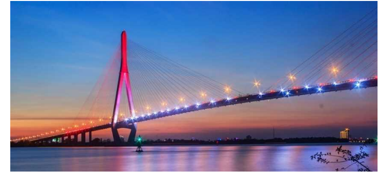
Can Tho Bridge (2010)
